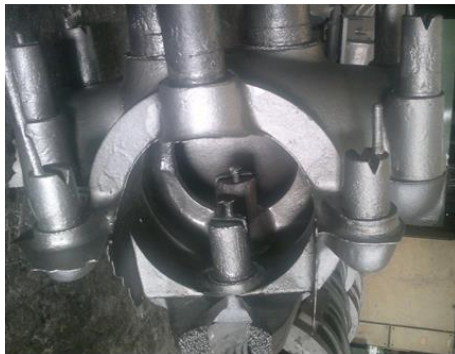
Figure 21: Runner broken through filters. No by-pass
